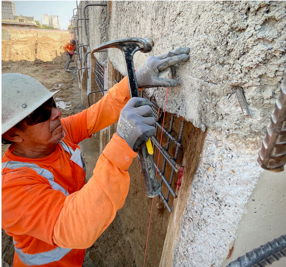
Esteban Casia working on Tulare Street
